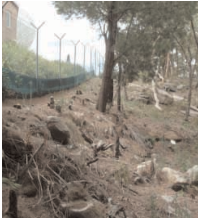
Vegetation clearance at Belrose Earth Station after cultural heritage investigations
