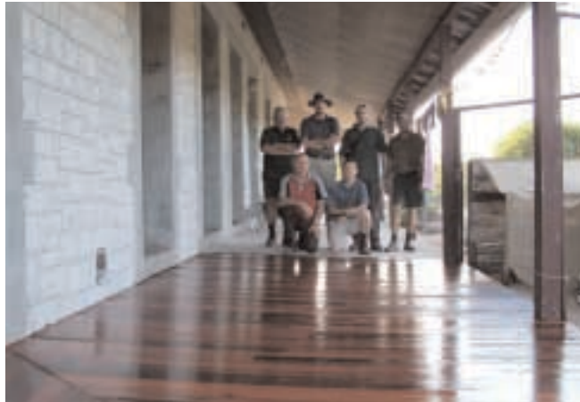
Verandah restoration at the old telegraph station, Nuytsland Reserve, WA
