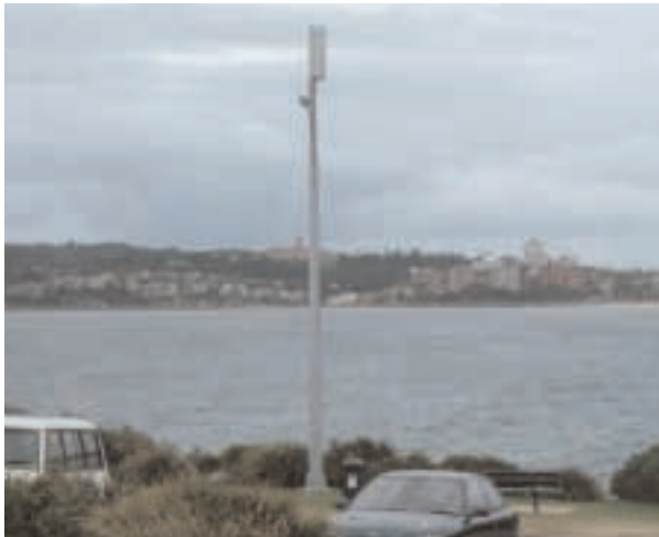
Integrated light pole and antenna support at Harbord, NSW
