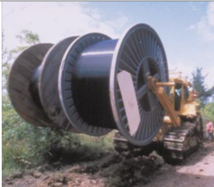
Fibre optic cable laying
