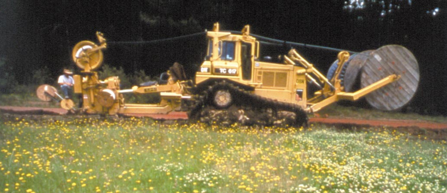
Fibre optic cable laying in rural areas
