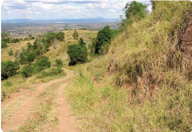
Track up Mount Stradbroke, QLD in the vicinity of the planned Optus underground cable installation.
