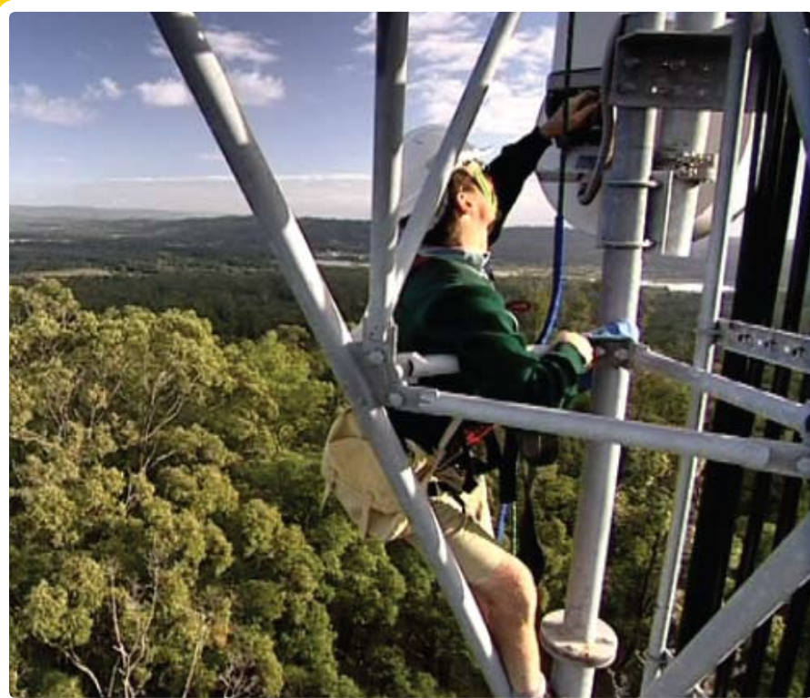
Optus technician working on a mobile GSM base-station.
